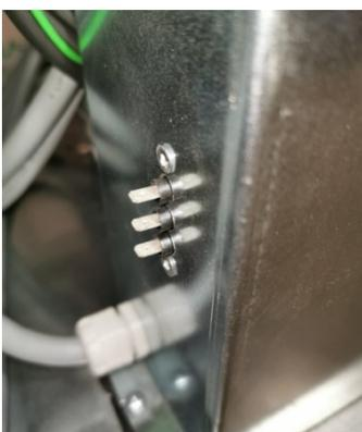
These units are equipped with a remote alarm plug for the connection to a remote alarm network.
